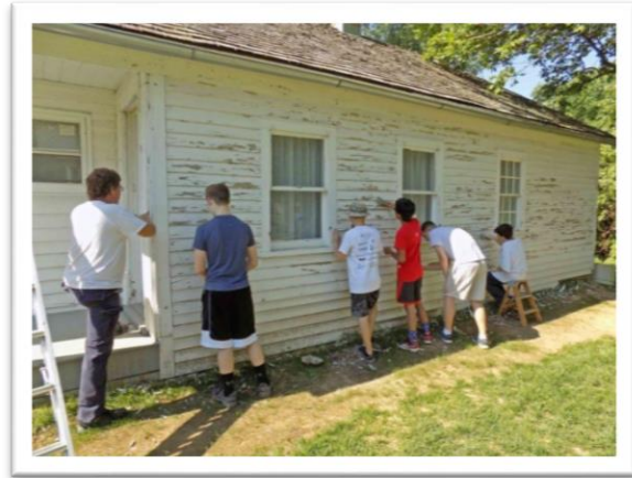
Scouts working on the Todd house, July 1, 2017
